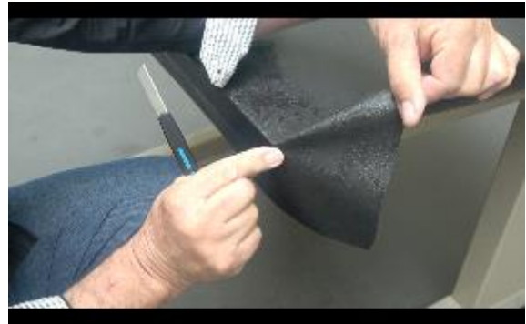
Rub the film 0.5cm around the corner..
